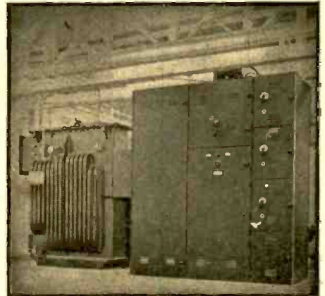
Sealed ignitron rectifier of factory-assembled load-center unit-substation type, installed in a large war plant. 300-kw, 250-v size.
